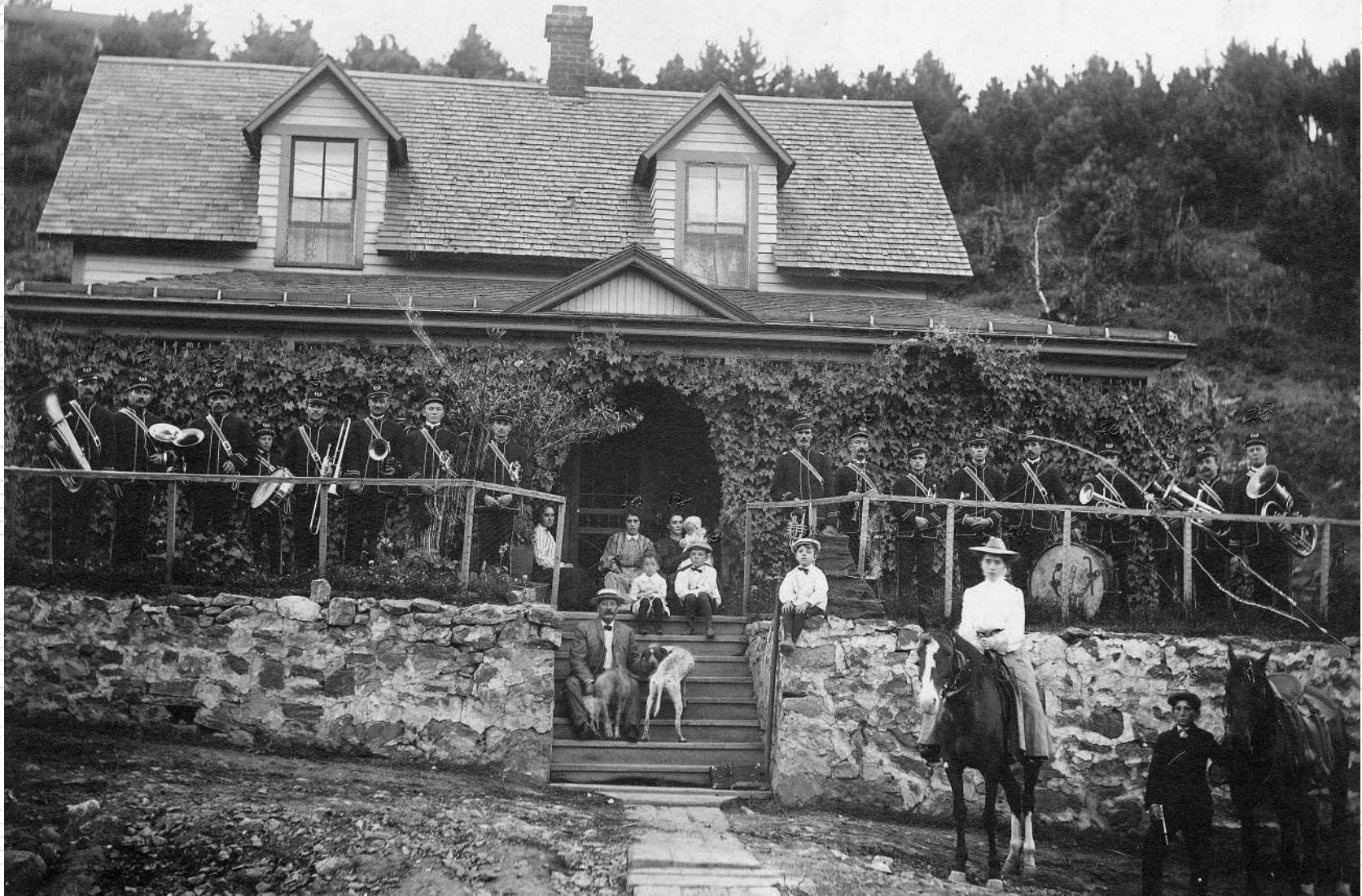
The Ancient Order of United Workman Band (Lodge 31) on the porch of the Blackford home in Terry in the summer of 1905. According to the identification on the photograph, those pictured, starting on the far left side of the porch, are: James Rhodda, Baptista Ornio, John Fountane, Fred Hart, Unknown, Harry Bennett, Matt Anderson, Sam Tretheway, Blackford daughter, Blackford daughter, Mrs. John Blackford, Blackford son, Dewey Black, John Blackford, Richard Chapman, Joe Cotti, Ed Mallette, Tom Thretheway, Jack Moon, John Hocking, John Grub, Bill Osborn, Unknown Jeweler, Blackford daughter and Chauneey Markham.
